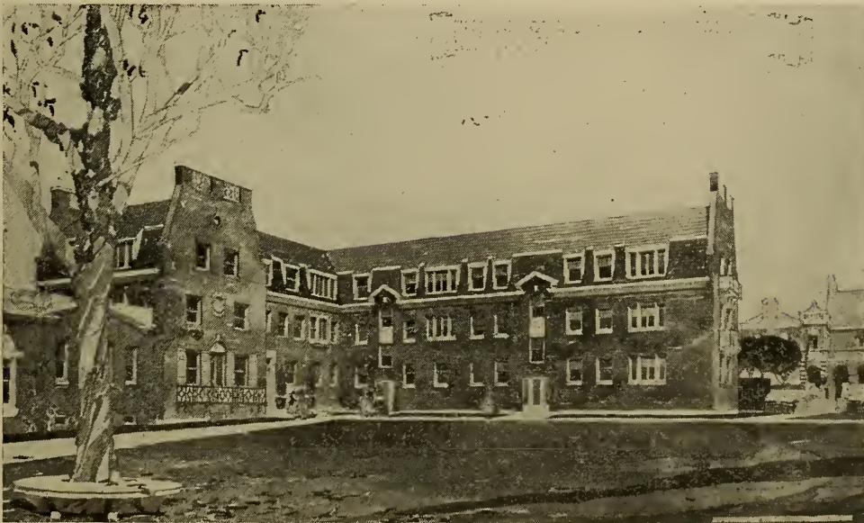
Architect's drawing of the new girl's dormitory. This building, now in course of construction, will provide residence for about 89 girls. It is, of course, entirely modern, comfortable and suitably appointed for the convenience of the women students who will make it their home. The new dormitory is adjacent to the old one—Mary Spiller.
